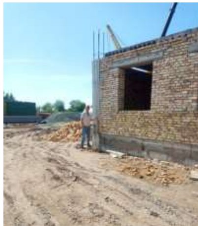
Figure 3. Measurement of building settlement after the installation of first-floor floor slabs (May 2024)
