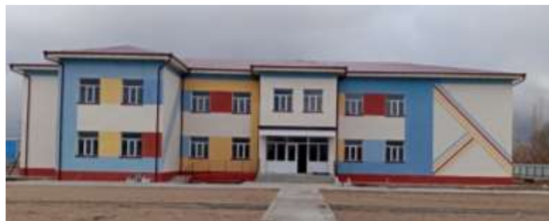
Figure 1. Overview of the building where subsidence observations were made
